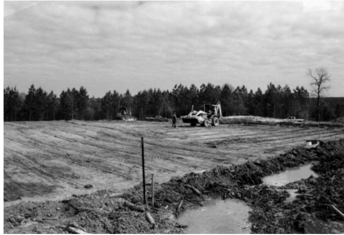
Figure 3-2. Bulldozer and backhoe-scraping in Area VIII.
