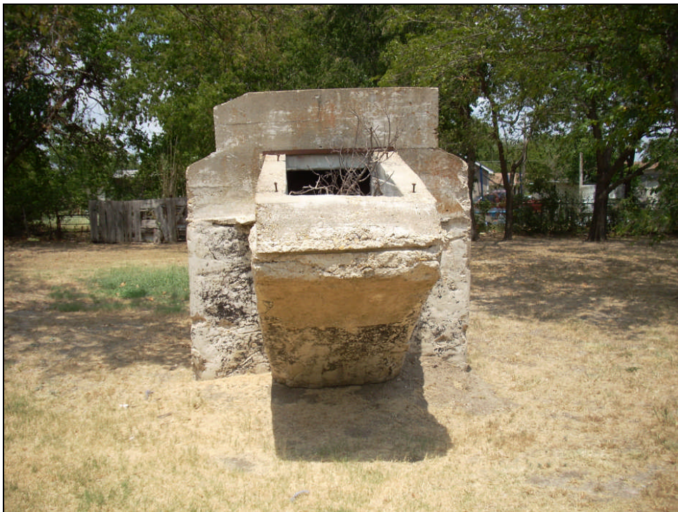
Figure 1. The front of the storm cellar. View is to the north.
