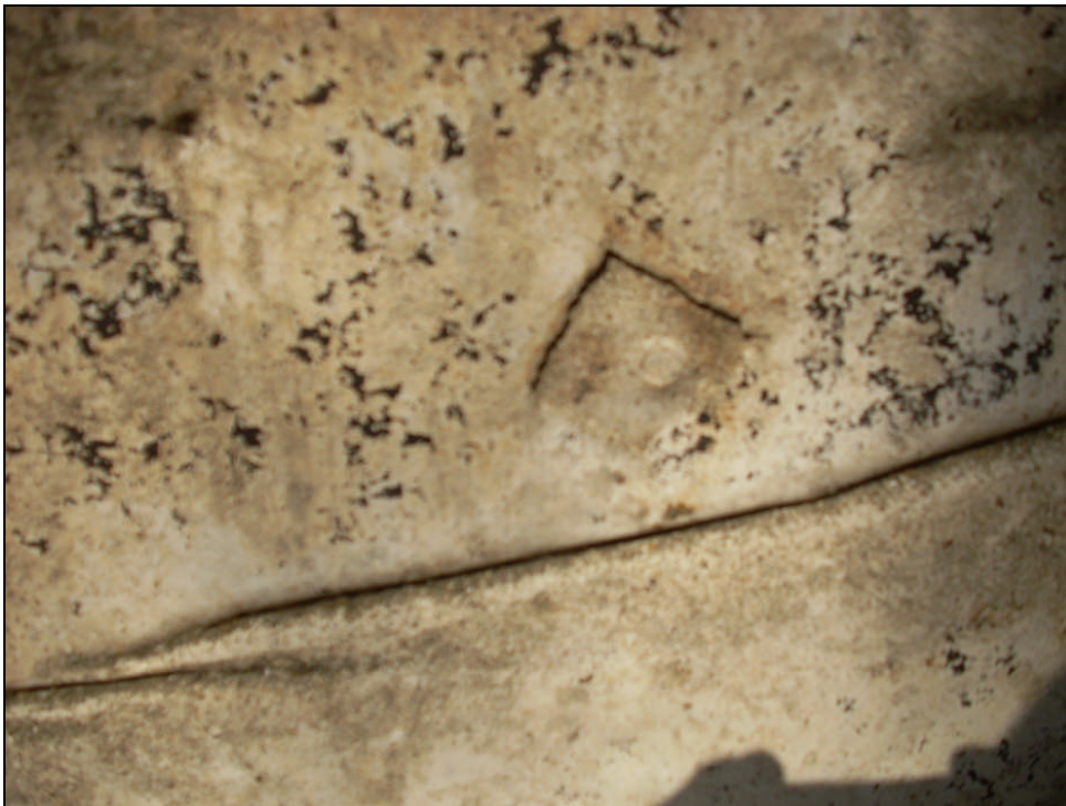
Figure 6. Diamond-shaped indentation in side of bottom portion of storm cellar.
