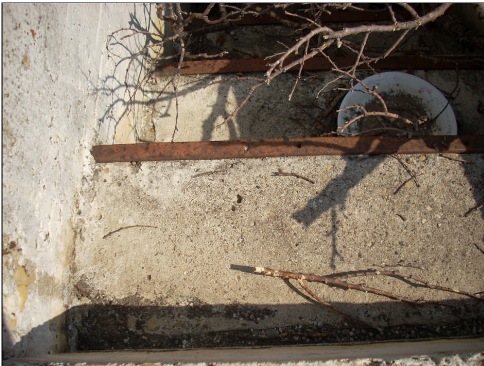
Figure 5. Steps leading into the storm cellar.
