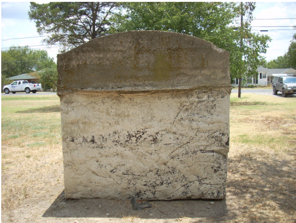
Figure 3. Rear of the storm cellar. View is to the south.
