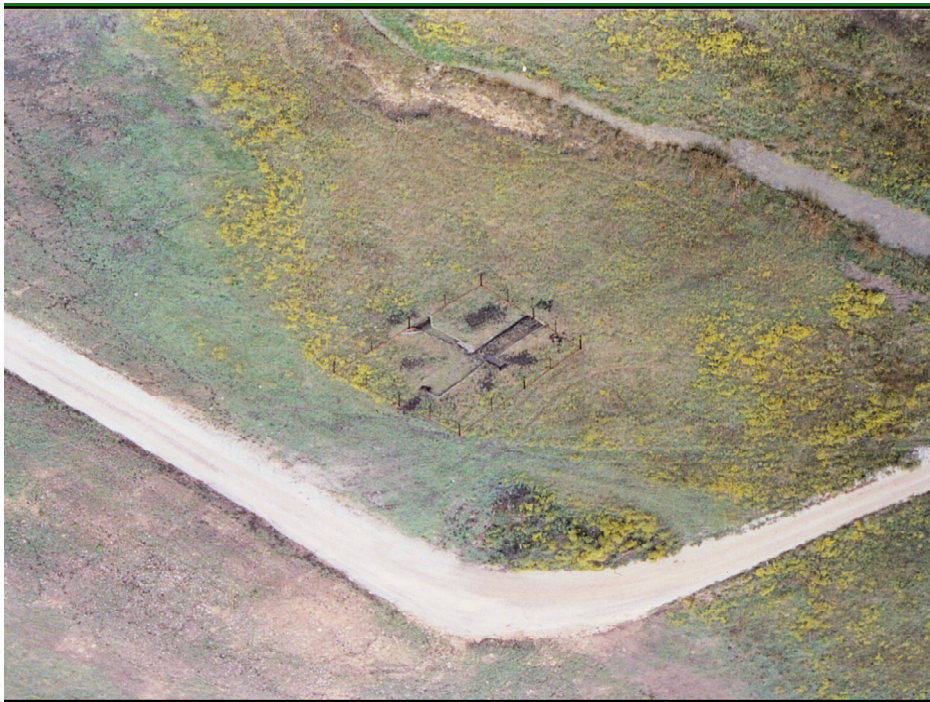
Figure 5. Aerial view of the Reinburg target near Hicks Field showing the pipe fence that has been built around the structure.
