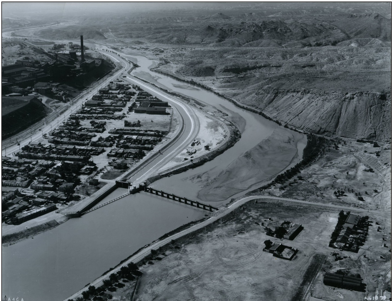
Smelertown and American Dam and Canal, August 18, 1939, looking southeast.
